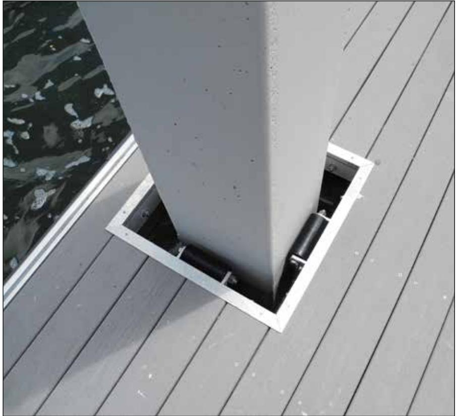
*A pile guide in a hybrid aluminum-timber dock.*
